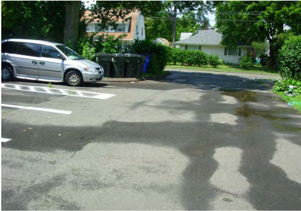
1. Parking area surfaces with some ponding, cracking
