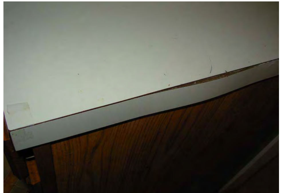
20. Countertop delamination at kitchens
