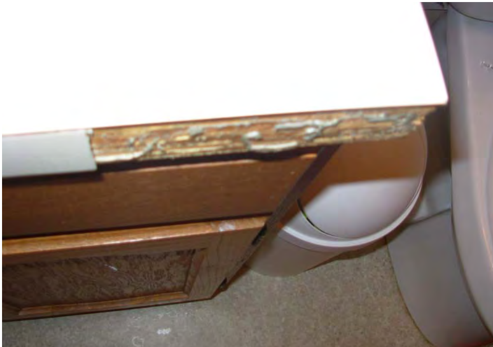
17. Vanity damage and delamination
