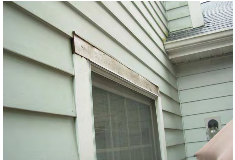
12. Poor trim repairs performed
