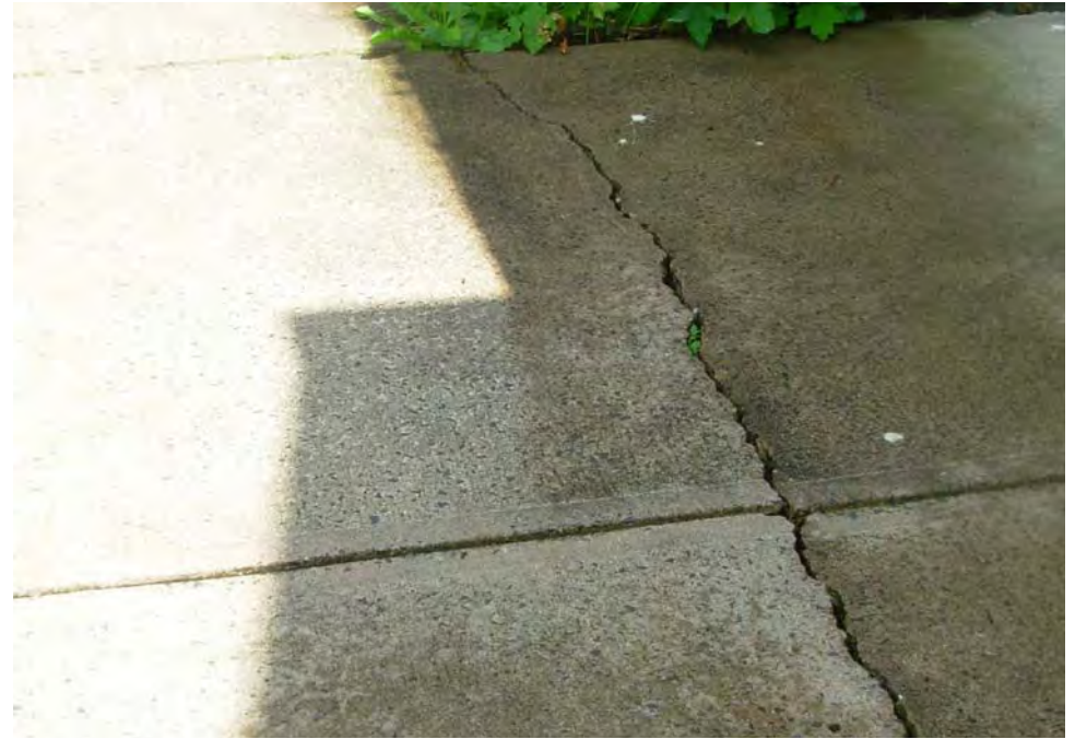
2. Concrete walkway cracking at front of building
