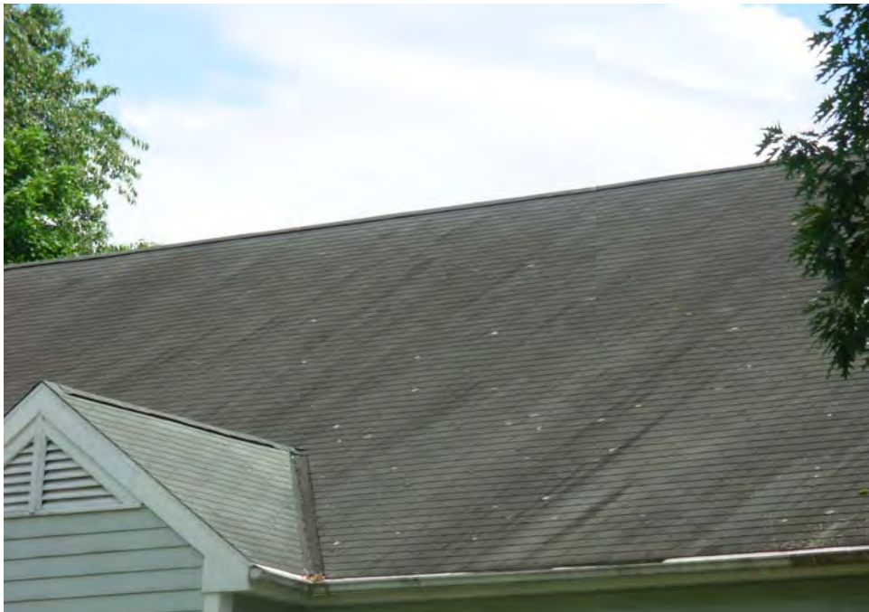
13. Original roofing shingles display organic growth and lifting
