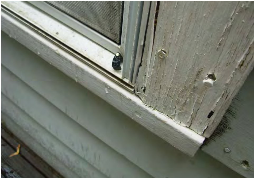
11. Spot siding and trim deterioration
